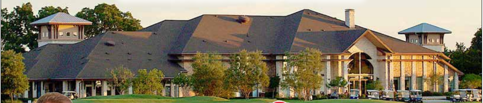
Heritage Ranch Clubhouse
