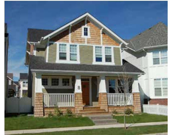
+ Proper articulation creates shadow lines, adds a sense of depth and creates a good streetface.
