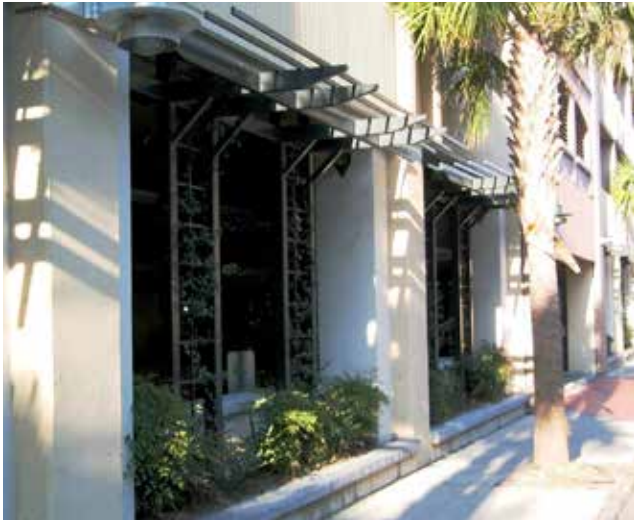
+ MODERN EXPRESSION. Metal arbors - not traditional awnings - can help add ornamentation to buildings as banal as parking garages.
