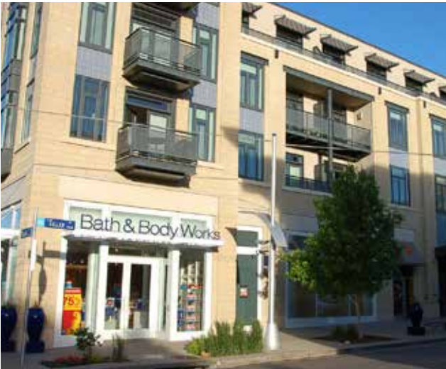
+ BASE, MIDDLE AND TOP ARTICULATION. The base of the building is one story tall and is clearly expressed through a change in the vertical plane toward the interior.
