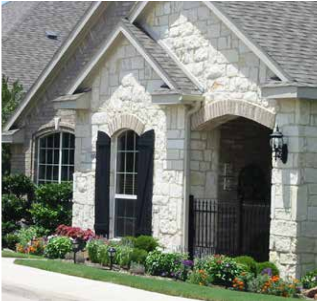
+ Shutters match the window shape and size.
