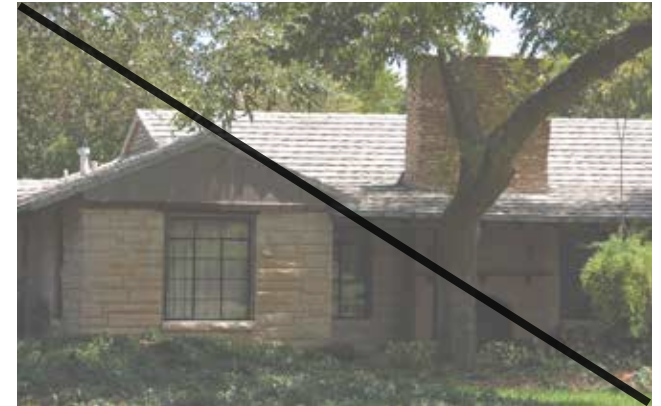
+ Metal simulated shakes do not relate to the scale of the building and appear fake.
