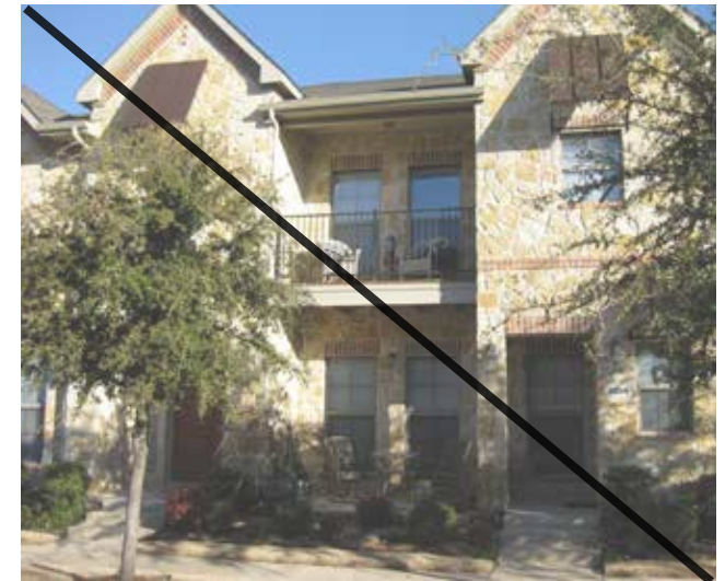
+ Casings do not meet the 3 1/2” requirement.
