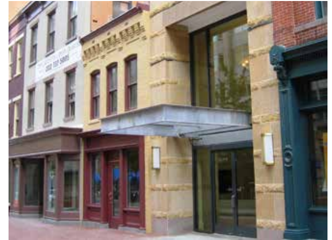
+ AWNING STRUCTURE AND MATERIALS. Cantilevered from a heavy stone base, this awning provides a simple and strong solution to inclement weather for this entry.
