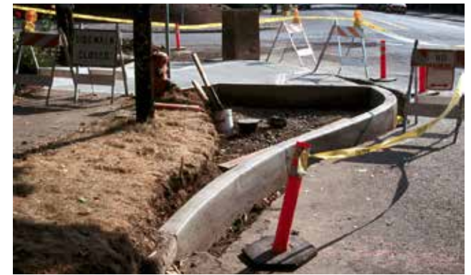
Constructing a Curb Extension, www.pedbikeimages.org/ Dan Burden
