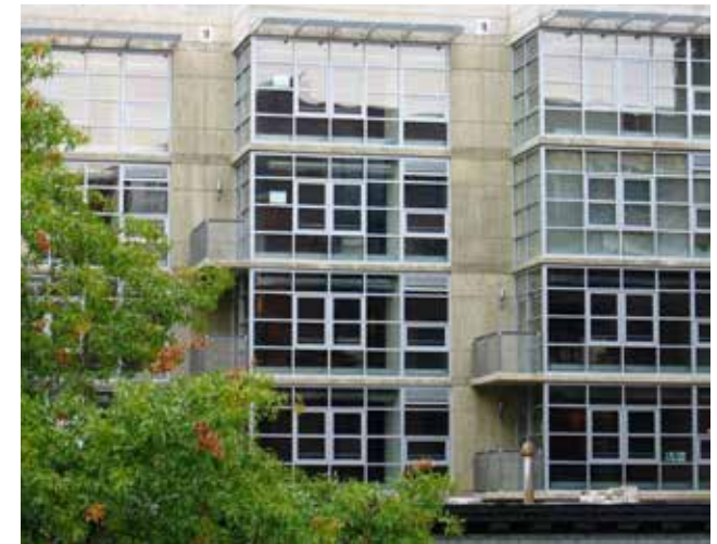
+ WINDOWS OF LARGER BUILDINGS. Windows in a wall of fixed lites permit modern facades and natural ventilation.
