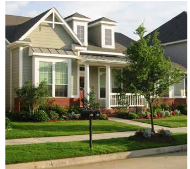
+ Casings are greater than 3 1/2” and the style of the windows match the building style.
