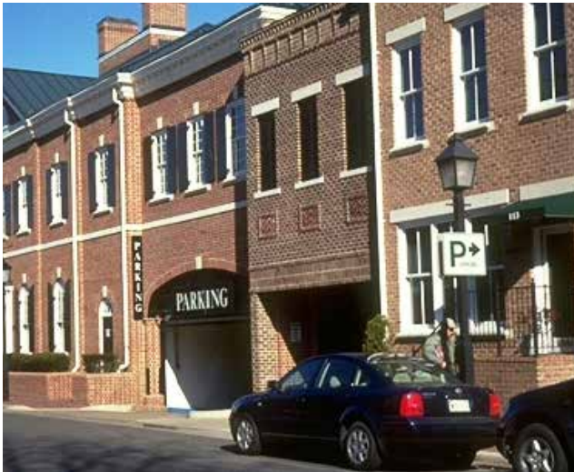
+ PARKING STRUCTURE FENESTRATION. Entrances to parking garages should be incorporated into the building facade to provide a seamless frontage along the street.
