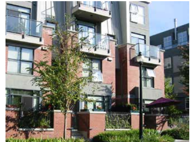
+ LIGHTER MATERIALS ABOVE HEAVIER. This building has a base (the lower two floors) rendered in brick with a variety of materials above. This illustrates proper materials configuration.
