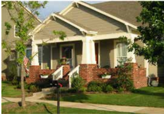
+ Just three materials (not including foundation) provides simplicity and elegance.
