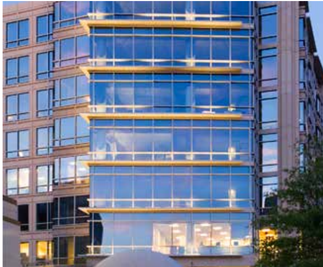
+ BUILDING WALL MATERIALS. Larger buildings may be clad in a variety of materials including curtain wall as an accent.
