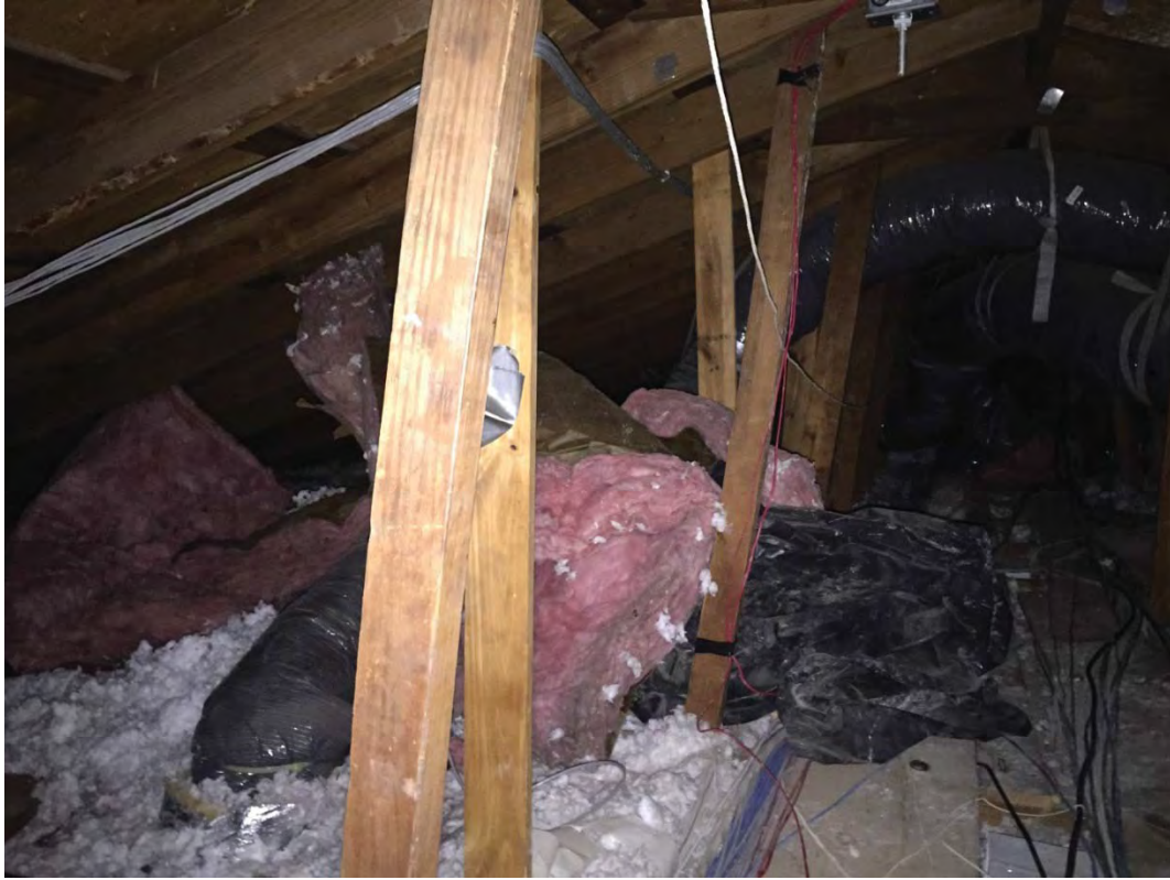
Photo S9. Ceiling Suspension Framing – Original 1960's Module
