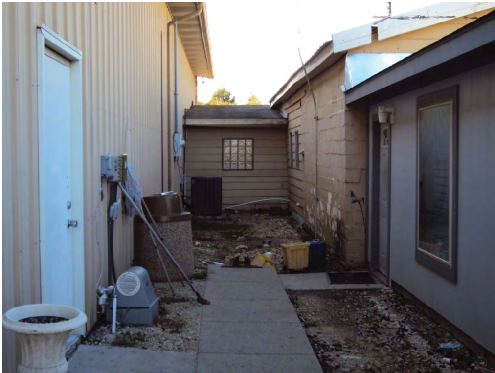
Photo A2. Building Additions
