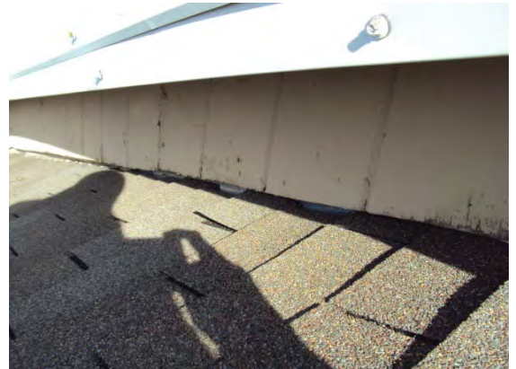
Photo A7. Roof Addition
