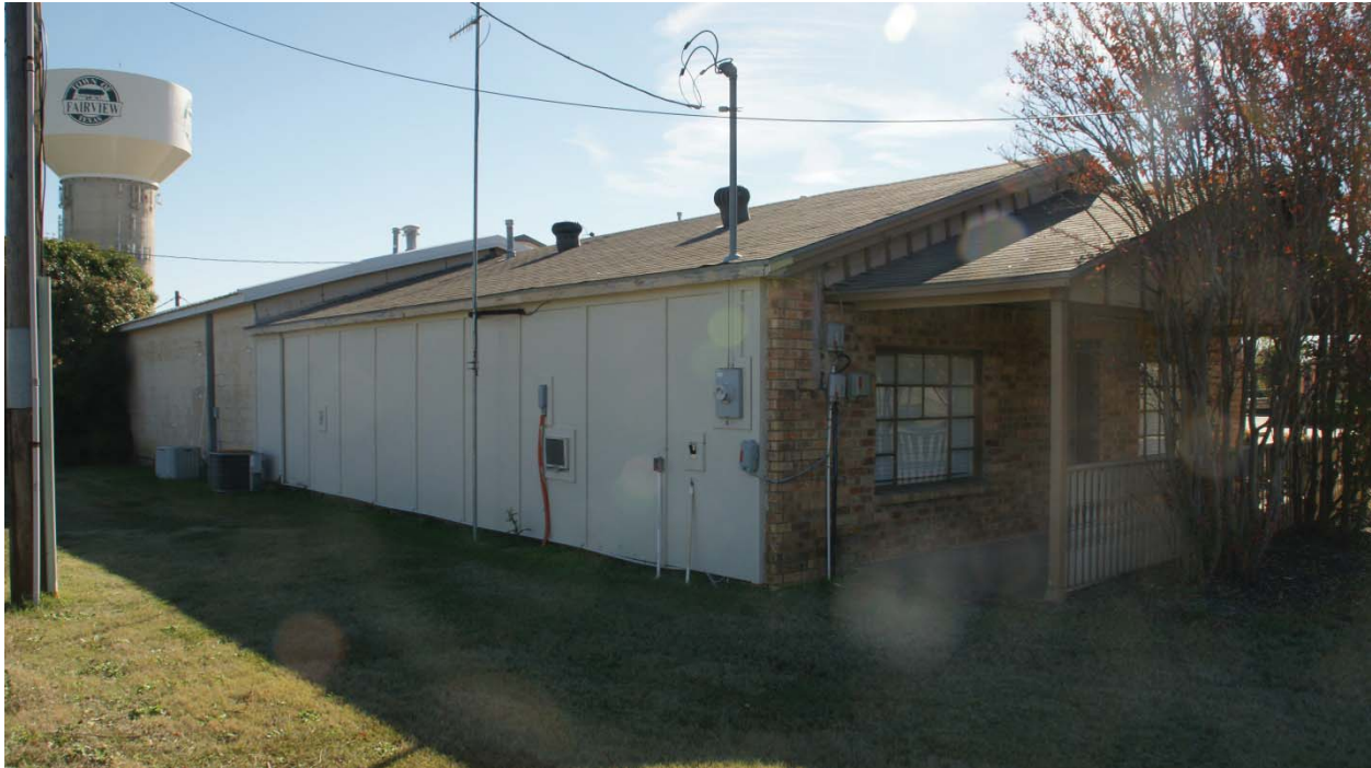
Photo S2. Northern Half of Roof, Trim, and Siding on 1960 Module
