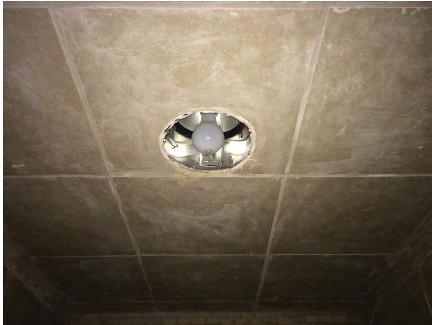
Photo E9. Fixture in Shower
