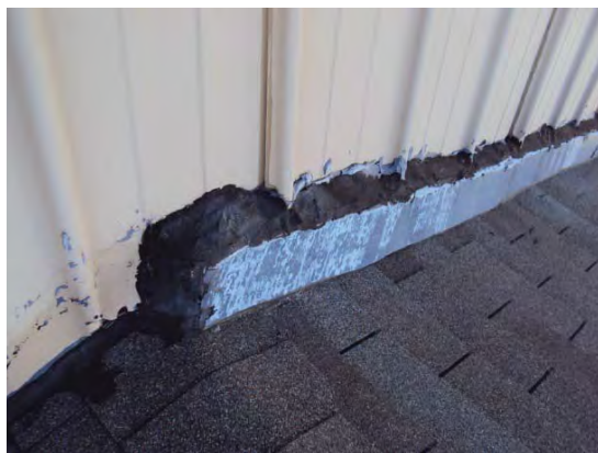
Photo A6. Roof Flashing
