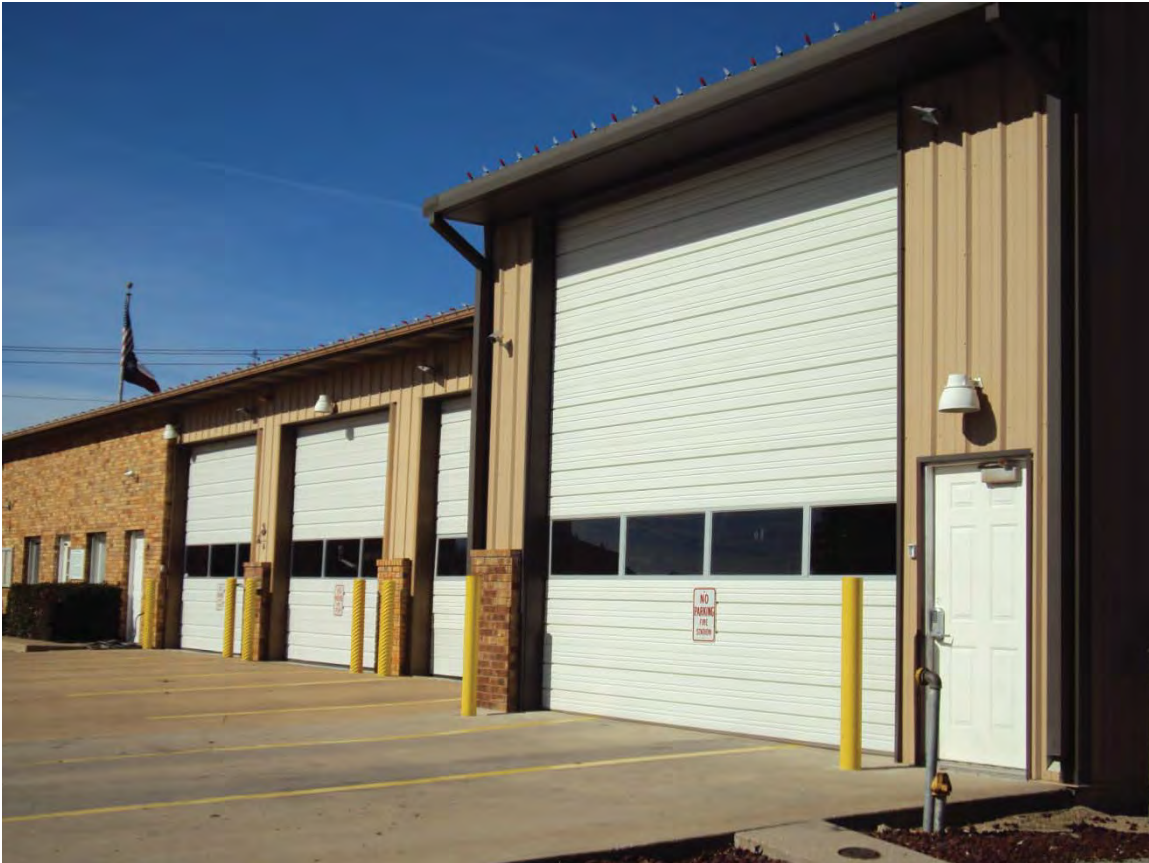
Photo A3. Apparatus Bays
