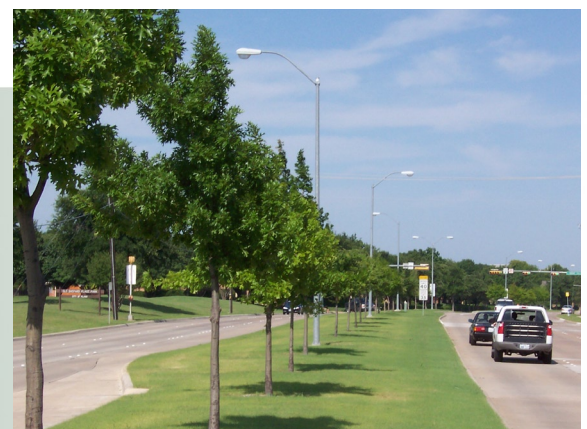
Six-Lane Divided Road
