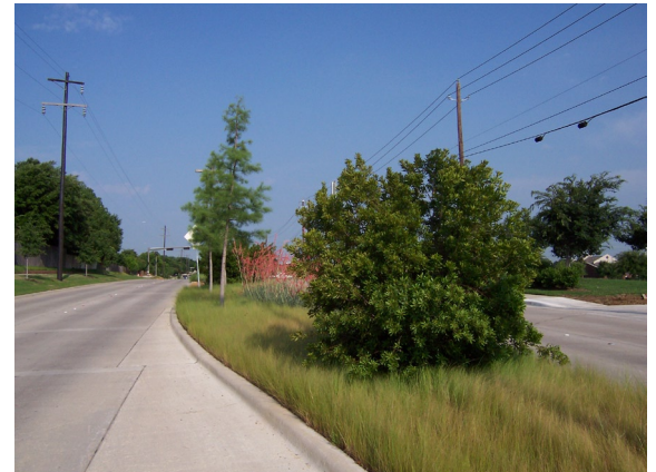
Four-Lane Divided Road
