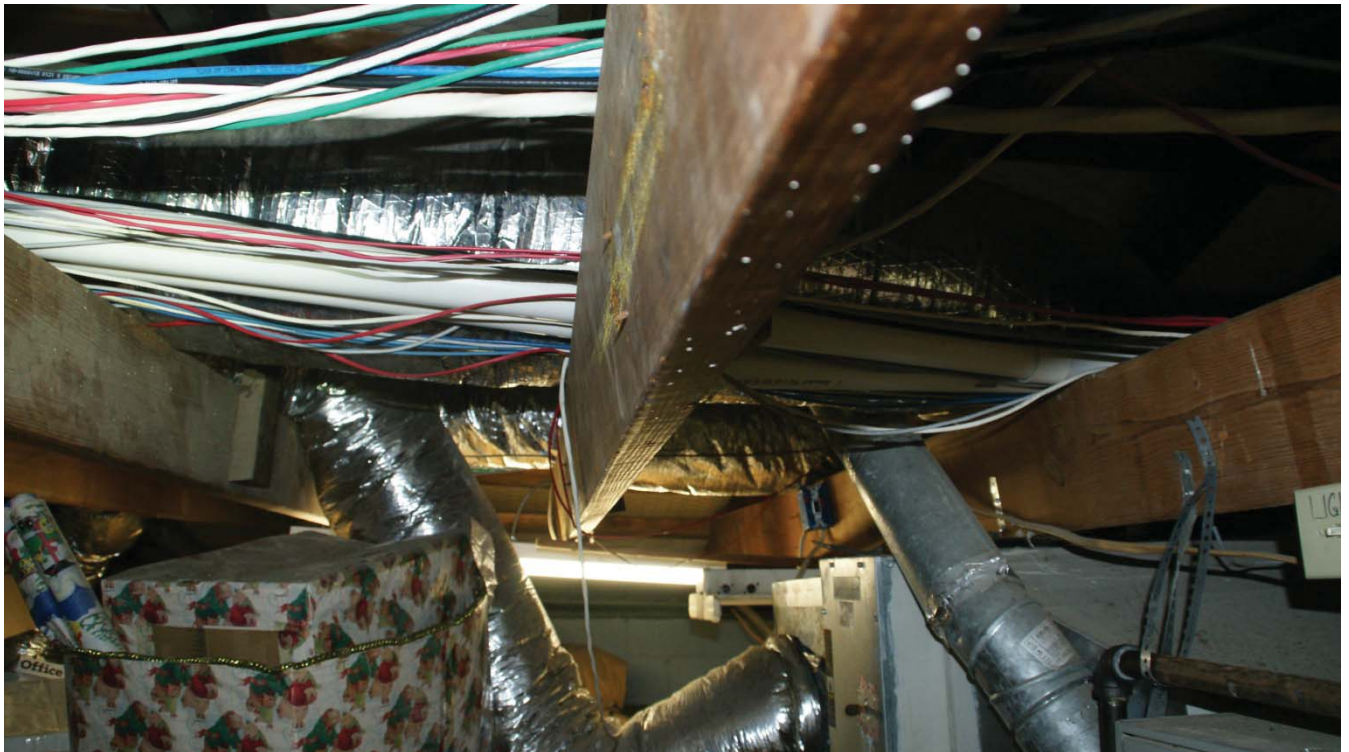
Photo S8. Twisted Bottom Tie
