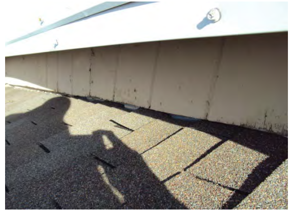
Photo A7. Roof Addition
