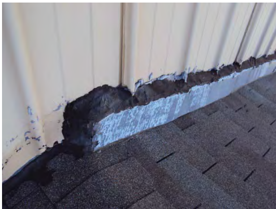
Photo A6. Roof Flashing
