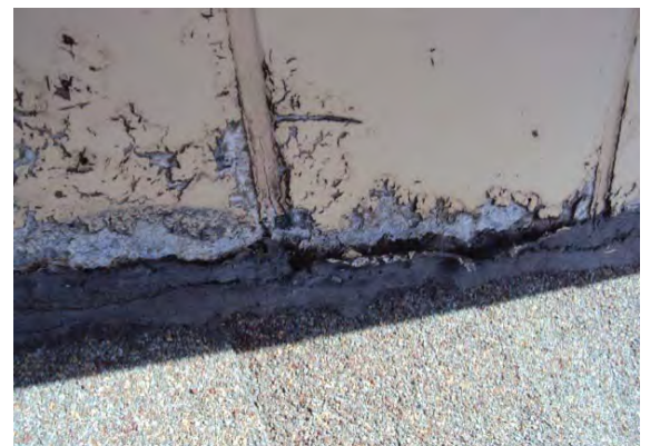
Photo A8. Deteriorating Sheathing
