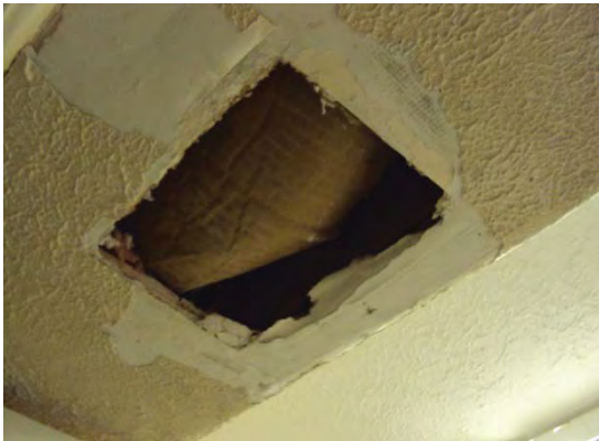
Photo A5. Roof Leak at Ceiling
