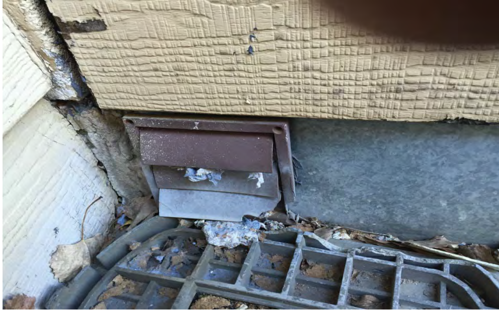
Photo M1. Clogged Dryer Exhaust Backdraft Damper
