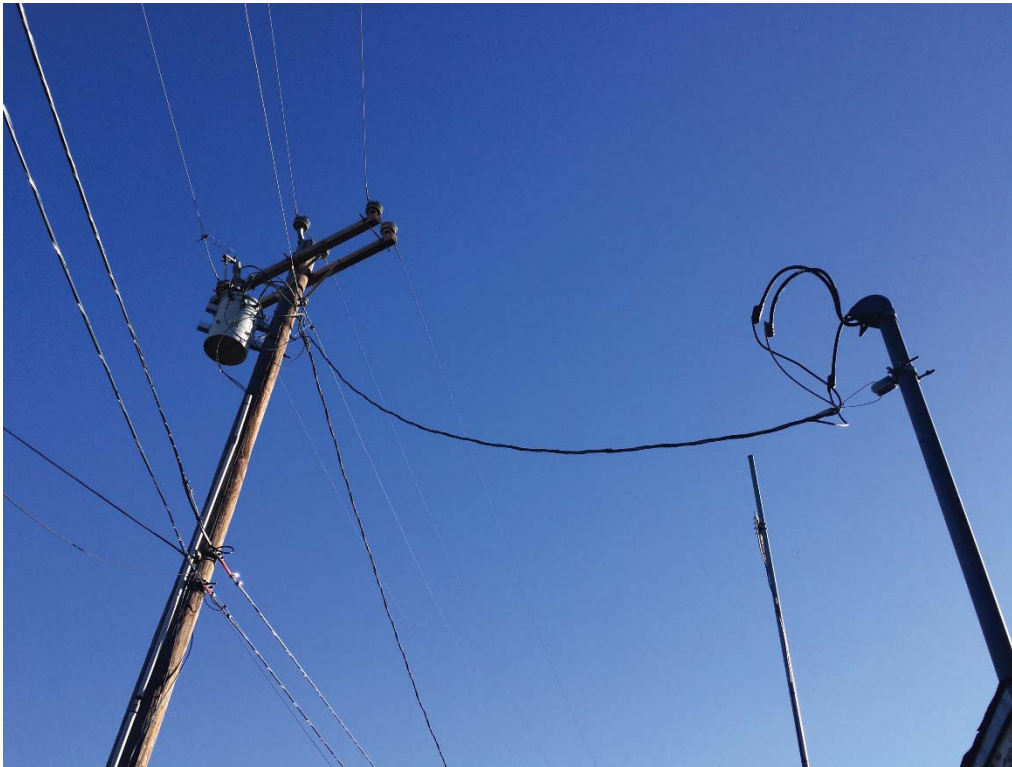
Photo E1. Overhead Service
