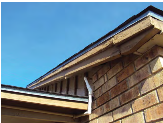
Photo A10. Wood Rake and Trim Rotting
