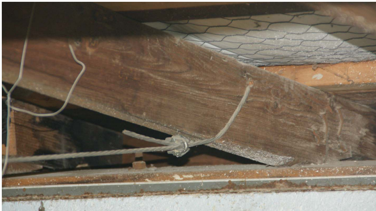
Photo S6. Cable Connection at Rafter
