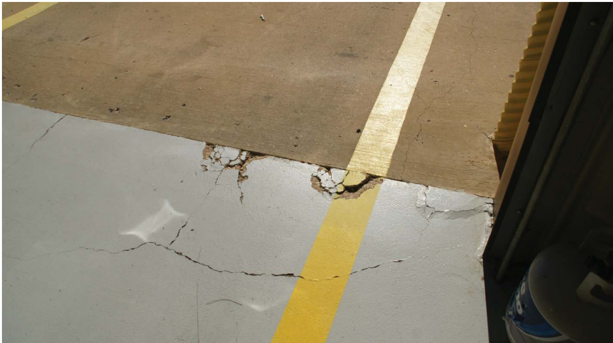
Photo S15. Edge of Slab Cracking Due to Wheel Loads at Vehicle Bays
