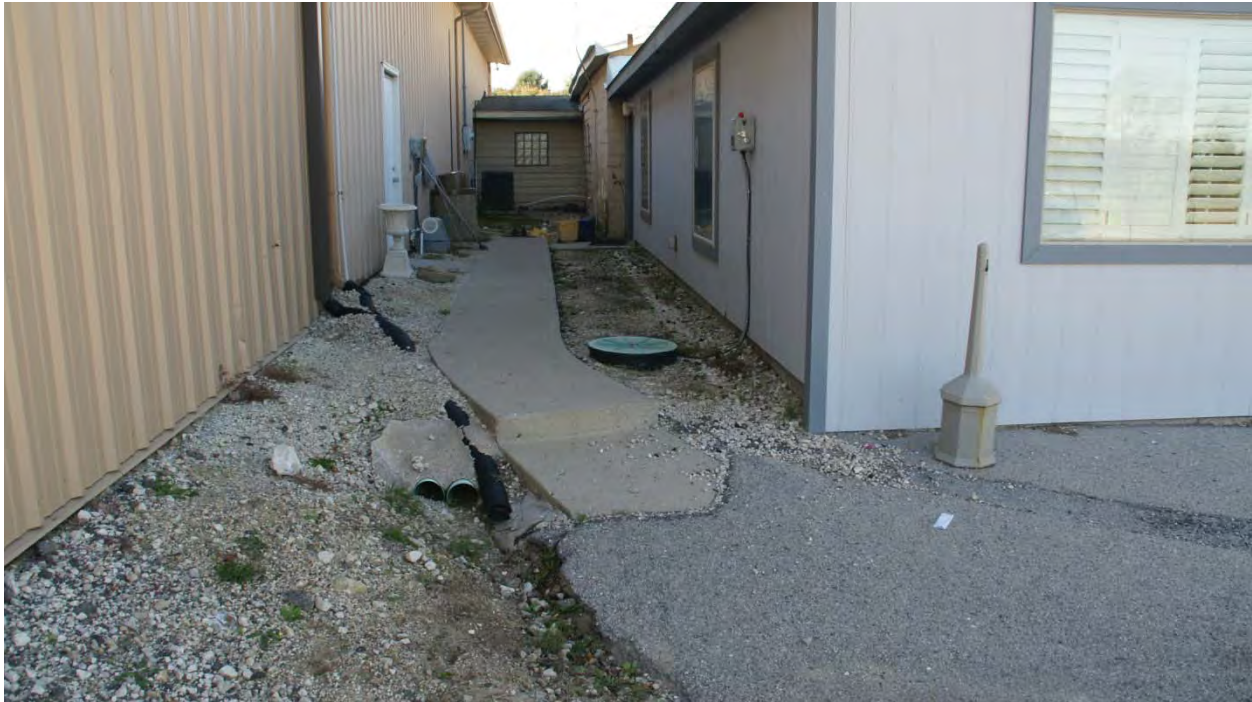
Photo S16. Area Between the North and South Wings
