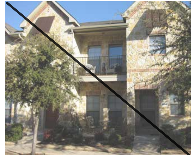
+ Casings do not meet the 3 1/2” requirement.
