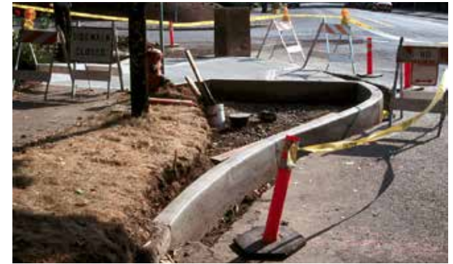
Constructing a Curb Extension, www.pedbikeimages.org/ Dan Burden
