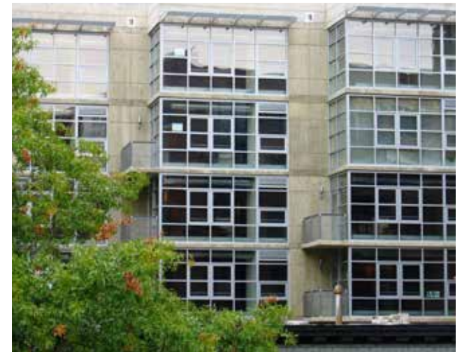
+ WINDOWS OF LARGER BUILDINGS. Windows in a wall of fixed lites permit modern facades and natural ventilation.
