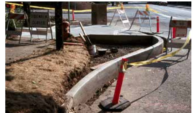
Constructing a Curb Extension, www.pedbikeimages.org/ Dan Burden
